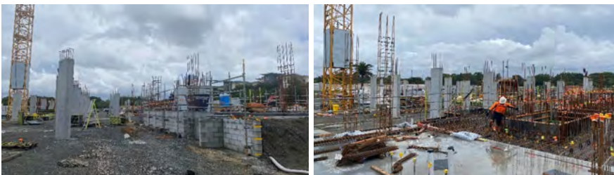
Onsite tower crane
